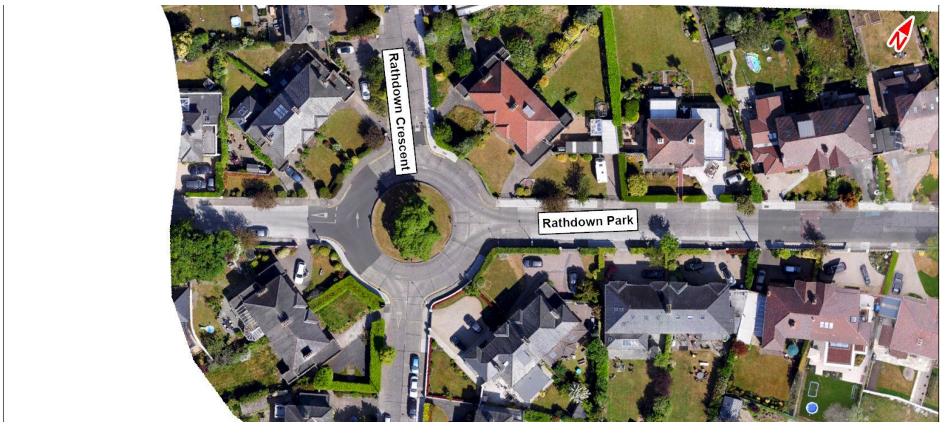
Image 6.7: Rathdown Crescent / Rathdown Park Roundabout
