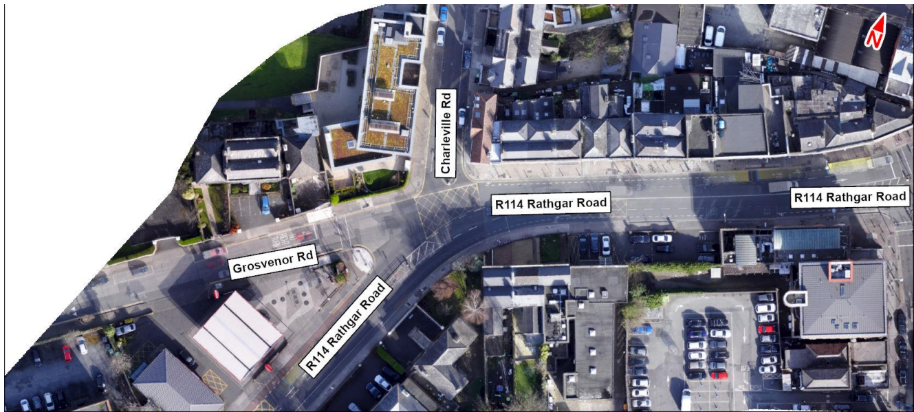
Image 6.18: R114 Rathgar Road / Grosvenor Road / Charleville Road Junction
