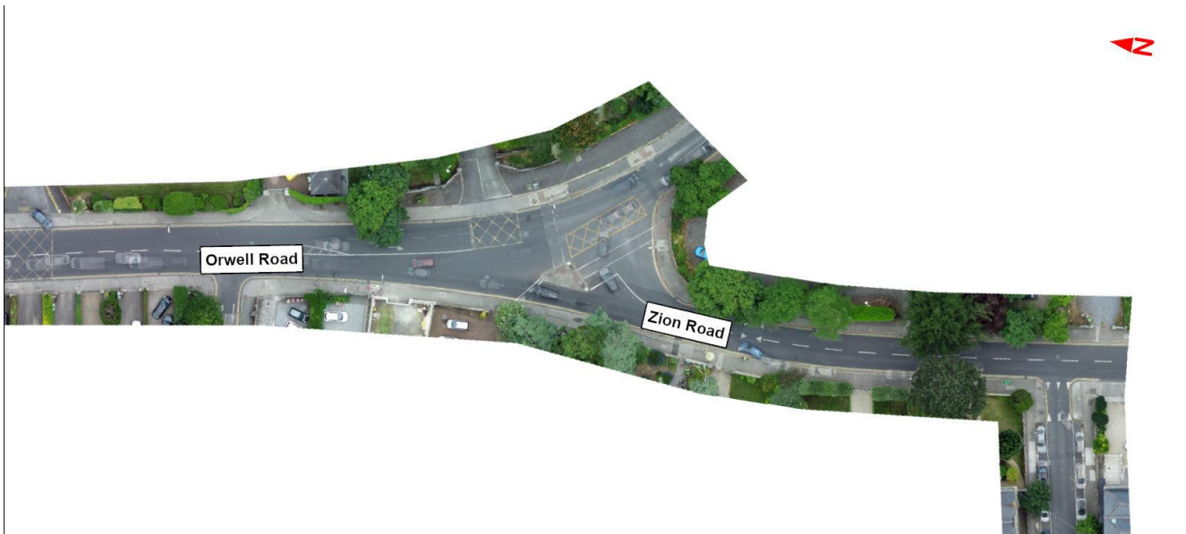
Image 6.15: Orwell Road / Zion Road Signalised Junction
