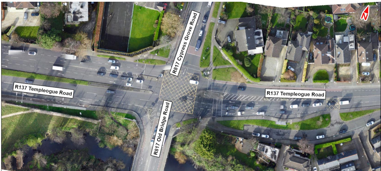
Image 6.2: R137 Templeogue Road / R817 Cypress Grove Road / Old Bridge Road Signalised Junction
