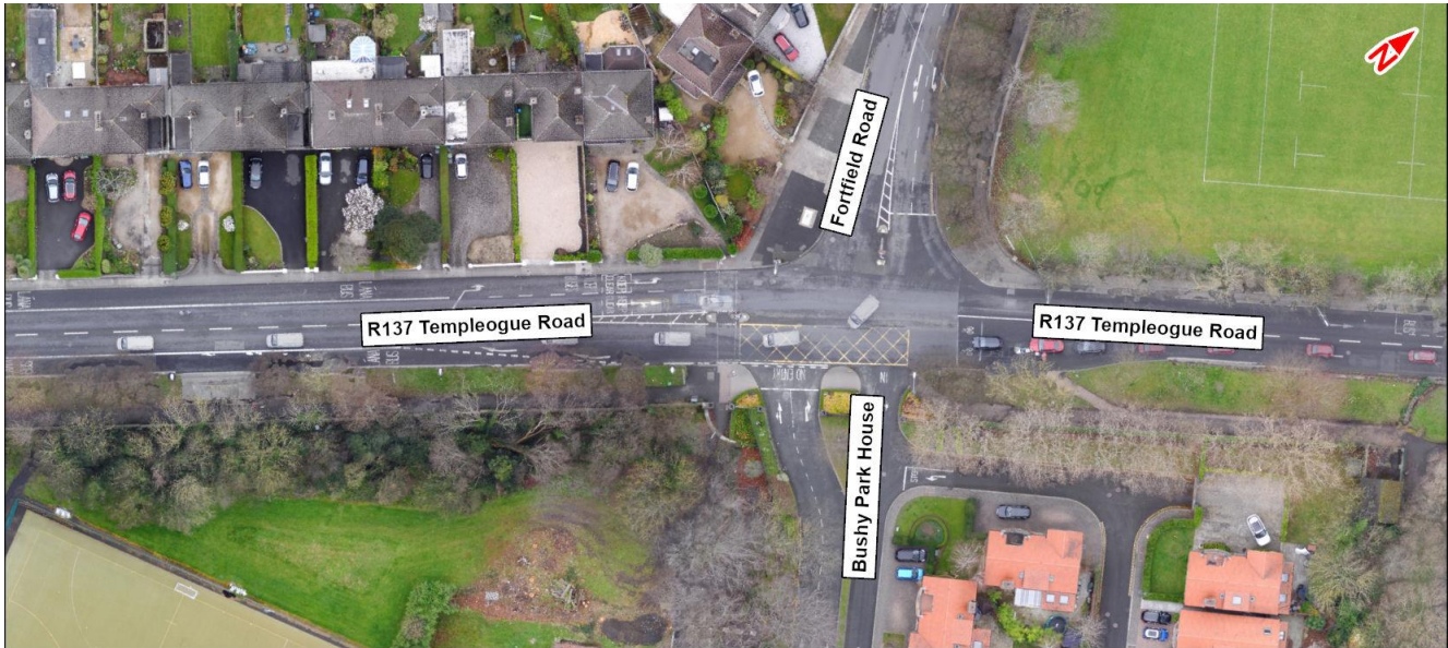
Image 6.4: R137 Templeogue Road / Fortfield Road / Bushy Park House Junction
