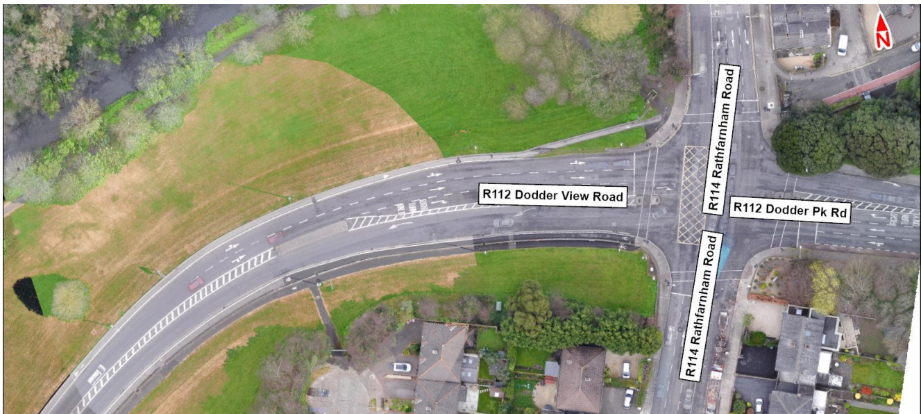
Image 6.12: R114 Rathfarnham Road / R112 Dodder Park Road / R112 Dodder View Road Junction
