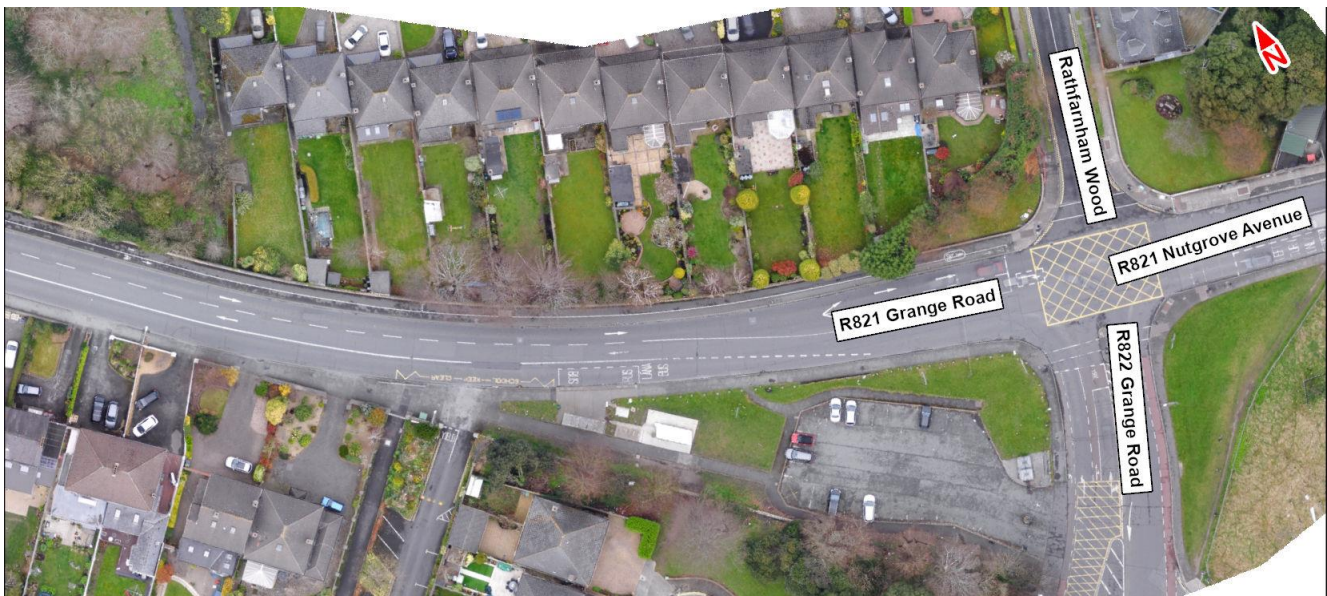
Image 6.8: R821 Grange Road / R821 Nutgrove Avenue / L8385 Rathfarnham Wood / R822 Grange Road Junction
