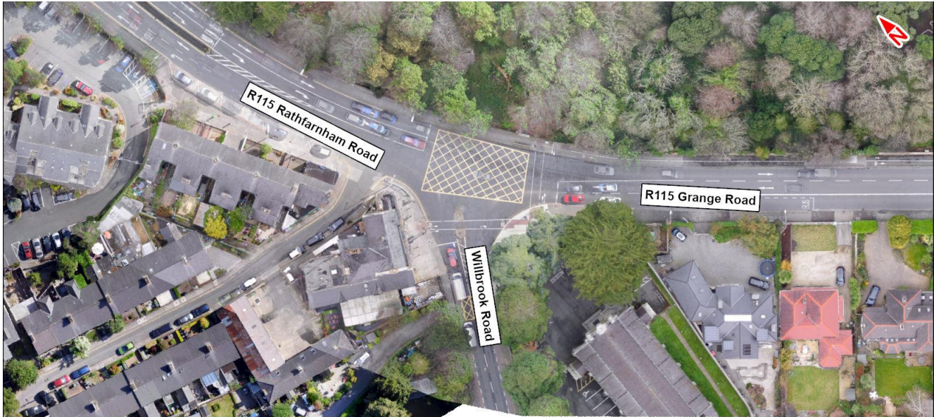
Image 6.9: R115 Rathfarnham Road / R115 Willbrook Road / R821 Grange Road Junction
